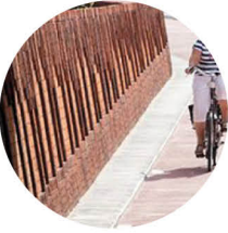
Bekleding tunnelwanden in baksteen Bron: https://www.wurck.nl/en/projecten/fietstunnels-doomsteeg-2/
